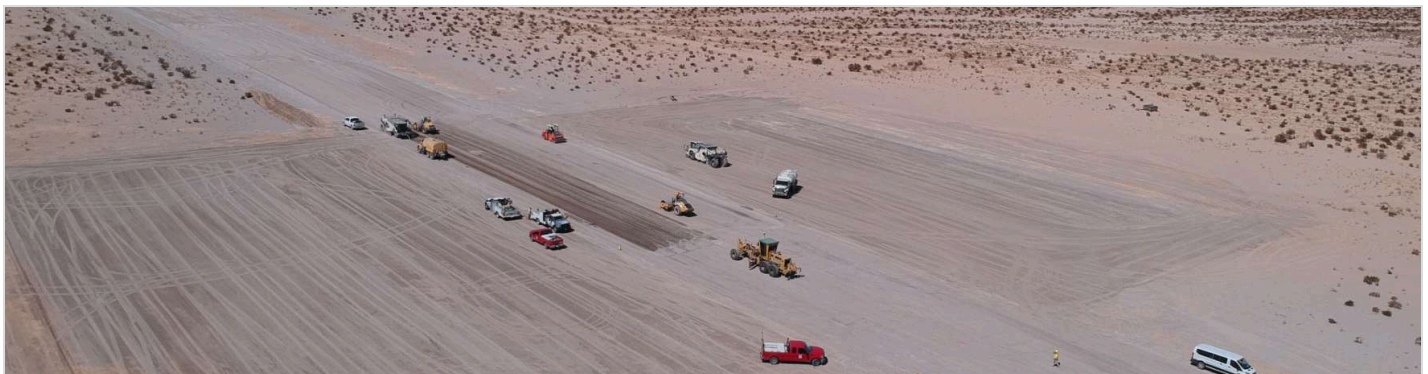
ALZ Sandhill military airfield, 29 Palms: LL-TEQ layer as the final wearing surface under aircraft loads.
