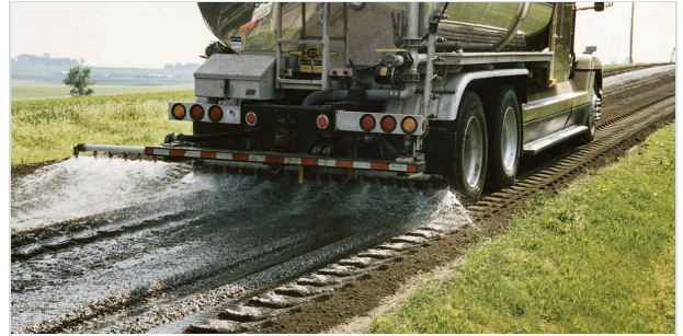
Distributor tanker truck with calibrated spray bar.
